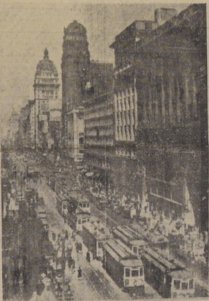
Market Street, principal avenida de San Francisco
